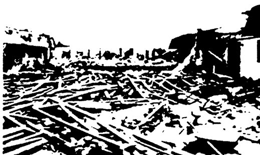
C-2. Upper left - Steel reinforced poured concrete tiebeam with steel roof straps exposed; upper right - streak of damage in senior citizen housing where tiebeams with roofs became airborne; lower left and lower right - Naranja Lakes complex where roofs acted similar to airplane wings lifting the roof and the tie beams off the buildings.
