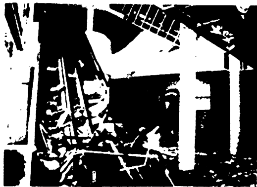
C-6 Burger King World Headquarters, showing significant external and internal views. Note that this well engineered building appeared to do well structurally. Although external walls and windows failed, the interior walls also failed. This is what mid-and high-rise condominiums will be learning the hard way. They should not be occupied during a hurricane unless there are hardened areas and were built to resist a potential storm surge.
