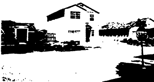
C-5. Upper left - CBS first floor, wood frame second floor; upper right - neighboring CBS both floors with concrete tie beams and tie columns - no failures of walls, but window and door failures; lower left - rebuild - replacing former wood frame second floor with CBS; lower right - new construction in Garden City, South Carolina. It should be noted that despite some "shoddy construction" in South Dade county, the great majority of the houses that were heavily damaged were still better built far better than the great majority of the homes along the Gulf of Mexico and Atlantic coasts from Texas through Maine.
