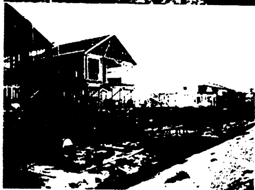
C-5. Upper left - CBS first floor, wood frame second floor; upper right - neighboring CBS both floors with concrete tie beams and tie columns - no failures of walls, but window and door failures; lower left - rebuild - replacing former wood frame second floor with CBS; lower right - new construction in Garden City, South Carolina. It should be noted that despite some "shoddy construction" in South Dade county, the great majority of the houses that were heavily damaged were still better built far better than the great majority of the homes along the Gulf of Mexico and Atlantic coasts from Texas through Maine.
