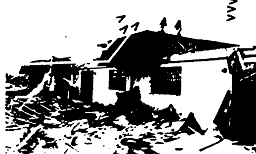
C-2. Upper left - Steel reinforced poured concrete tiebeam with steel roof straps exposed; upper right - streak of damage in senior citizen housing where tiebeams with roofs became airborne; lower left and lower right - Naranja Lakes complex where roofs acted similar to airplane wings lifting the roof and the tie beams off the buildings.
